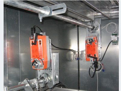
AIR HANDLER DAMPER ACTUATORS 22...1400 in-lb
