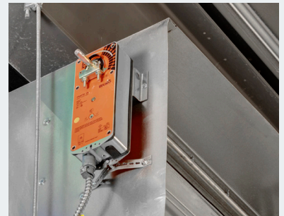
FIRE AND SMOKE DAMPER ACTUATORS 18...180 in-lb
